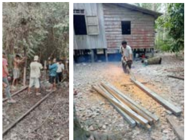
Our staff built the bridge in Jerumbun
